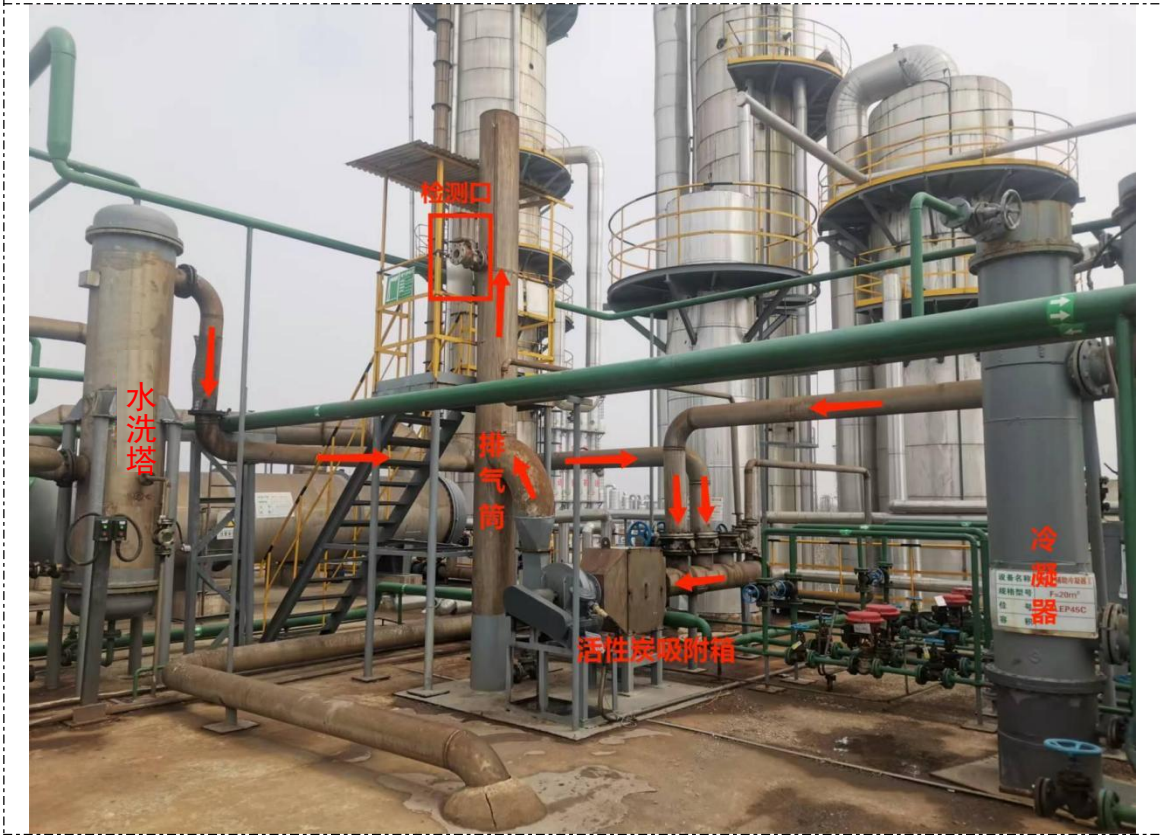
酒精蒸馏（南）不凝气、杂醇油不凝气冷凝+水洗+活性炭
